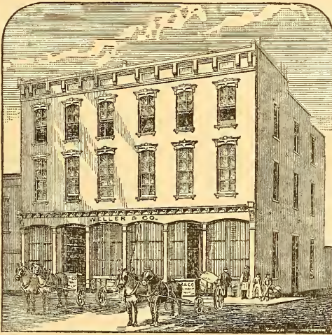
WELLER & CO.'S PEANUT FACTORY—WATER STREET.
